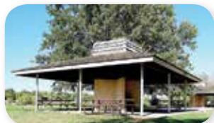
East Shelter House (A) West Shelter House (B)
